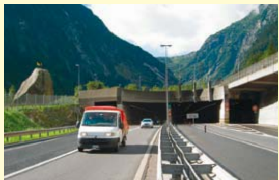
CLIC has proved itself in numerous road tunnels such as the Gotthard tunnel in Switzerland.
